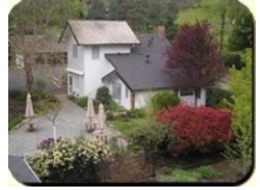
View of Carriage House from the 3rd Floor Mansion window
